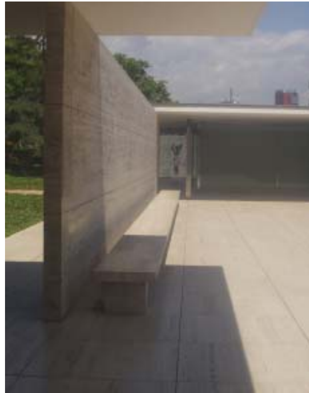
Mies van der Rohe's Barcelona Pavilion is experienced by moving through it but the devices it uses are classical and its understanding of space is, like its materials, neutral and passive
